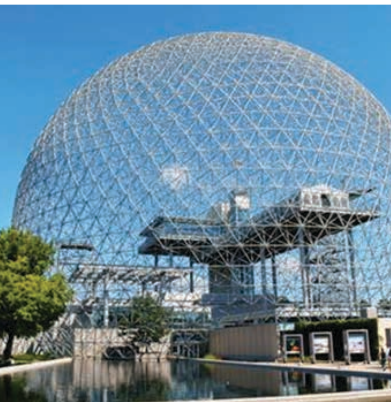
Figure 1 Buckminster Fuller geodesic dome, the USA pavilion in Montreal exhibition 1967, is a structure which was inspiration, as mimicry, to Kroto who named molecule C_{60} : fullerene. Icosahedron is composed of 20 triangles and Buckminster cupola is composed of 20 \times n triangles as optimization of design, mass and energy (light). (Wikipedia)
